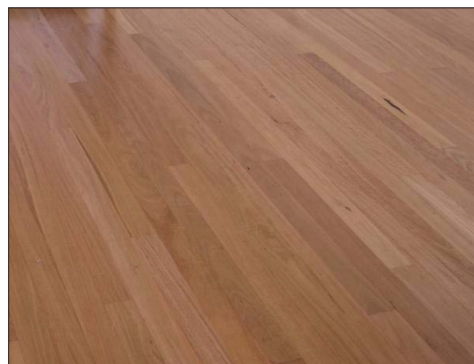
A select grade Blackbutt floor where the backsawn gum vein toward the top right exceeds grade limits but is acceptable within the floor.
